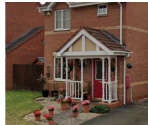
Door with wooden porch.
