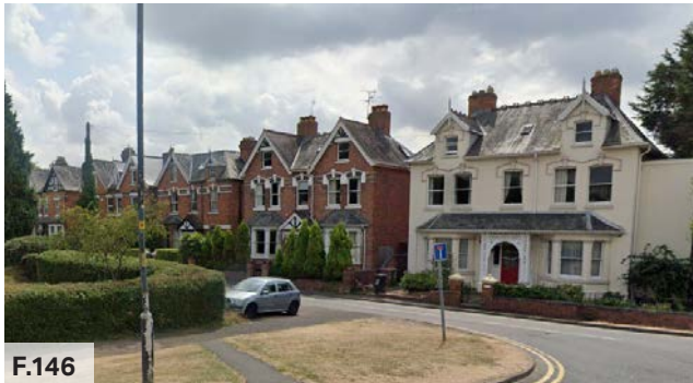
Figure 146: Roofline with slightly varied heights and roof pitches, shown on Ombersley Way with a mix of cross gable/hip roofs and dormers.
