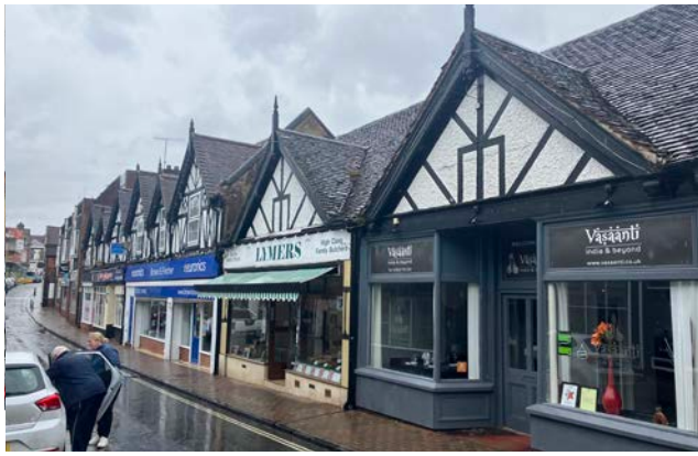
Figure 148: Uniform roofline with some variations in roof heights, shown on High Street with gable fronting roofs and decorative fascia.
